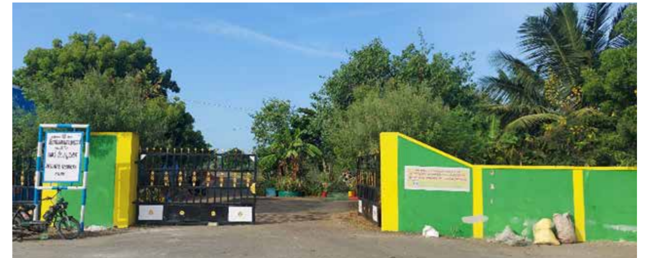
Figure 11: Resource Recovery Centre at Vadakadu
